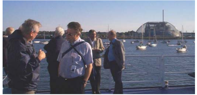
New household waste incinerator, guarded against seagulls by a giant stainless steel mesh canopy.
