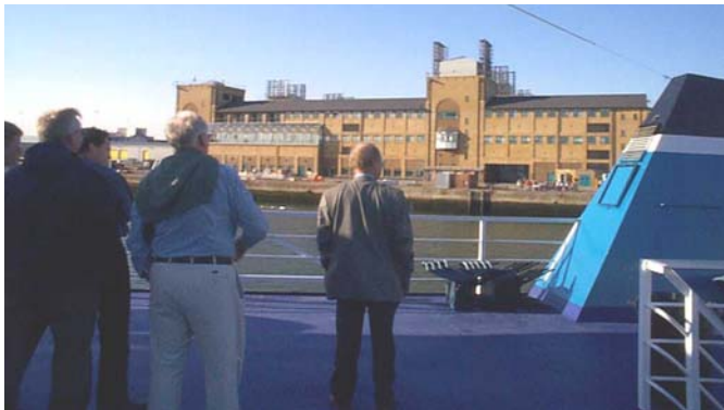
The new University Oceanography Centre, bristling with fume discharge stacks
